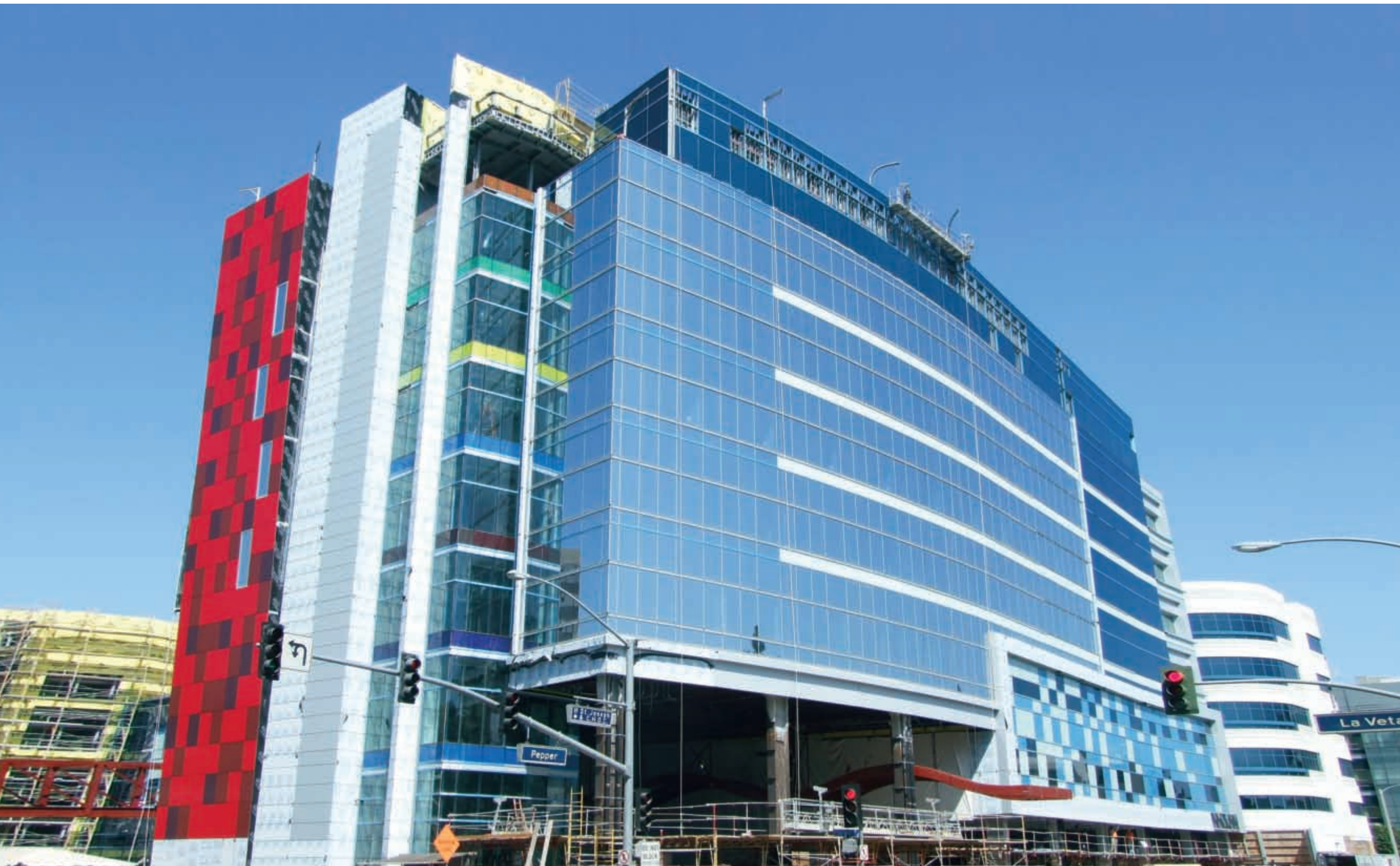
CHOC Children's new, state-of-the-art tower, at about 70 percent complete, August 2011.
